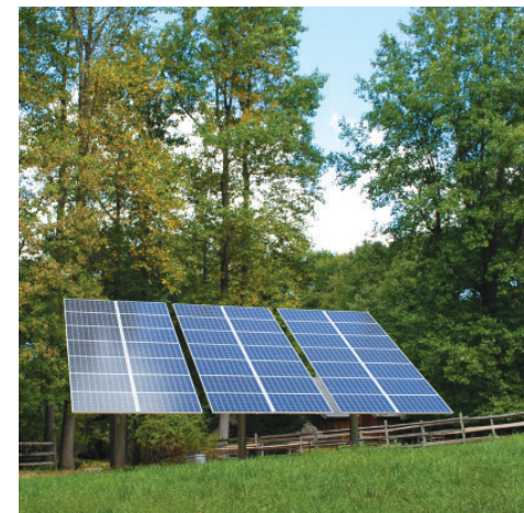
A 9.45 kW pole-mounted solar PV installation on a residential property.
